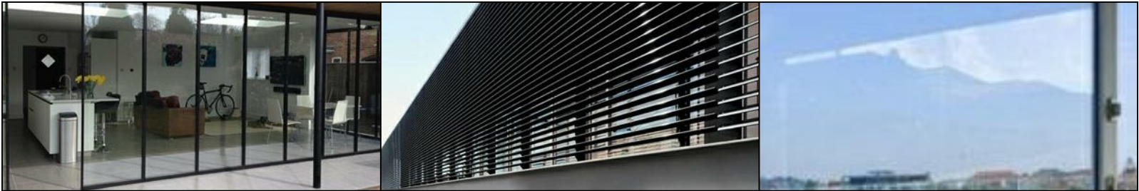
WF. WINDOW FRAMES COMMERCIAL GRADE ALUMINIUM MATTE BLACK OR SIMILAR SC. METAL SCREEN ALUMINIUM SCREEN MATTE BLACK GL. GLASS GLASS WINDOWS AND DOORS CLEAR GLASS *NOTE: WINDOWS AND DOORS ALSO SUBJECT TO BASIX REQUIREMENTS
