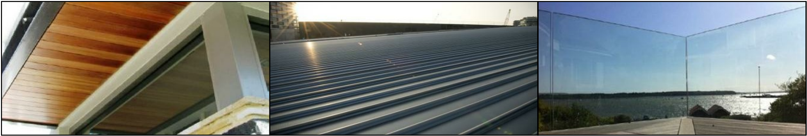
SO. SOFFIT TIMBER SOFFIT OR SIMILAR RO. ROOF KLIP-LOK MATTE BLACK OR SIMILAR GB. GLASS BALUSTRADE FRAMELESS GLASS
